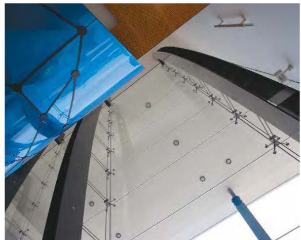
The combination of glass, steel, stainless steel and Duraliner™ fibre cement sheets, form a striking contrast between sophisticated building materials.
