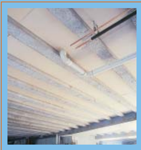
Underside of 'Ultrafloor' System showing essential services can be easily accessed through the Duraform™ sheets.
