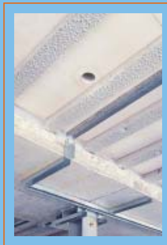
Underside of 'Ultrafloor' System showing essential services can be easily accessed through the Duraform™ sheets.
