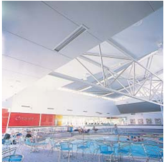
Kids' leisure pool ceiling lining and facade to Health & Fitness centre comprises 6.0mm Duralux™ fibre cement sheets
