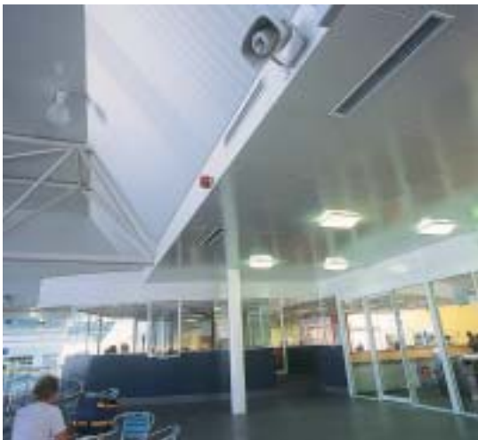
Duralux™ fibre cement sheets used for ceiling lining and facade of administration centre
