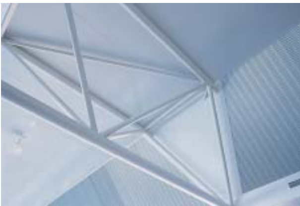
Detail of roof truss passing through the Duralux™ fibre cement sheets
