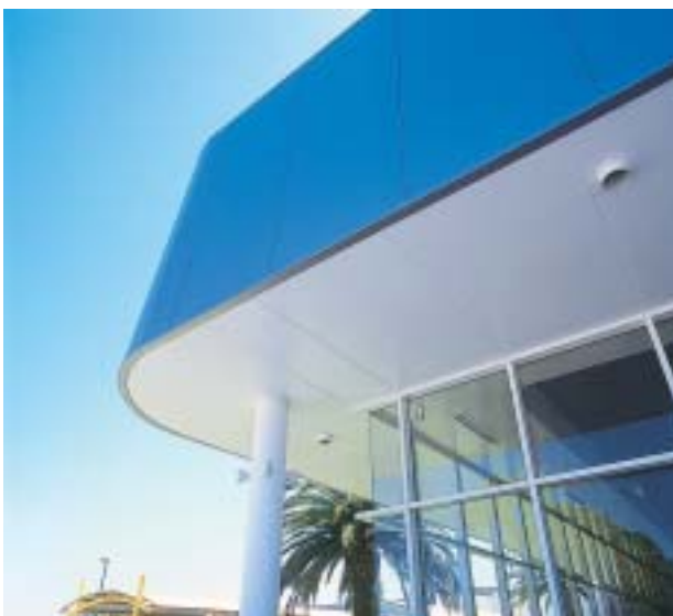
The smooth Duralux™ fibre cement sheets permitted a high standard of finish to be achieved to soffit linings and the entry.
