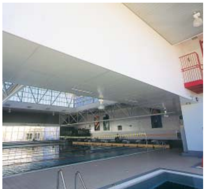
Bulkheads separating pool areas are clad with Duralux™ fibre cement sheets.
