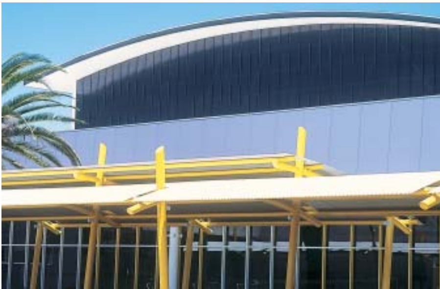
To aid ventilation to the main pool area, slotted BGC Duralux™ fibre cement sheets were used for soffit linings.
