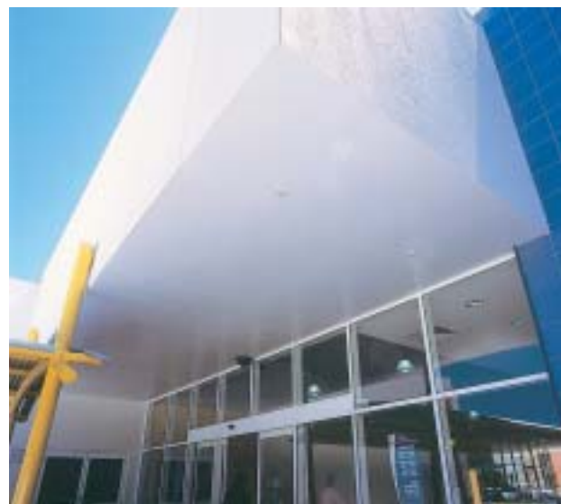
The smooth Duralux™ fibre cement sheets permitted a high standard of finish to be achieved to soffit linings and the entry.
